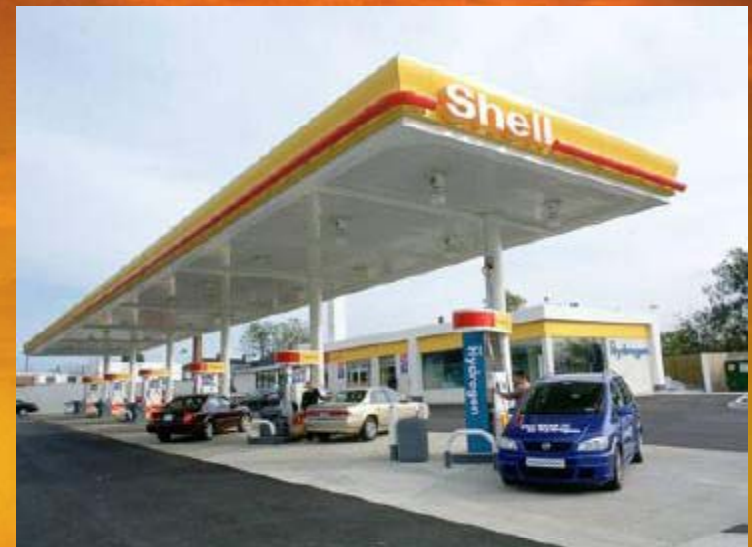
Shell H2 station in DC
