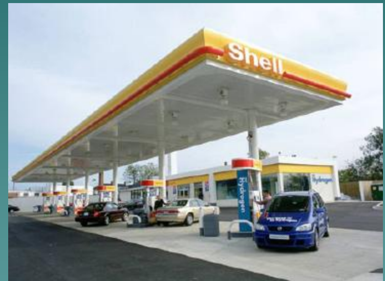
Shell H2 station in DC
